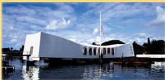
Rotary Club of Pearl Harbor www.pearlharborrotary.org
